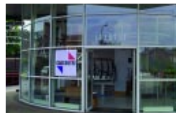
New offices at Altrincham
